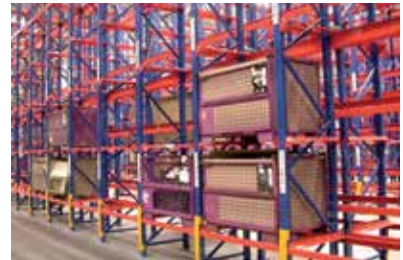
Open face racking
